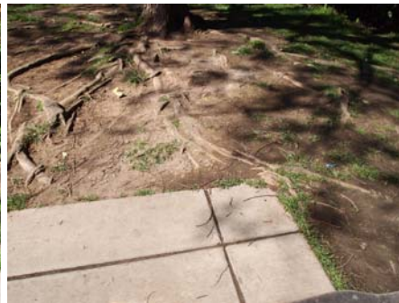
TREE ROOTS UPHEAVING PAVEMENT
