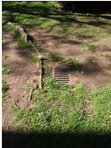
ROOTS DAMAGING CATCH BASIN
